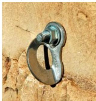
**Hardware:** climbing equipment placed in cracks or on faces to protect climbers from falling including chock, nuts, friends, pitons, and bolts.
